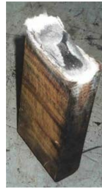
Fig. 3 – Blocking from Fig. 2 failure
